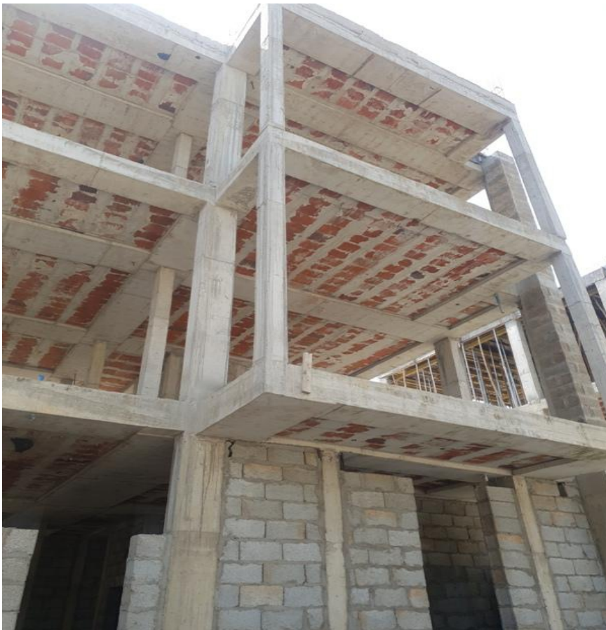
Concrete frame structure / 5 bedrooms Development on 4 floors at Guzape District, Abuja
