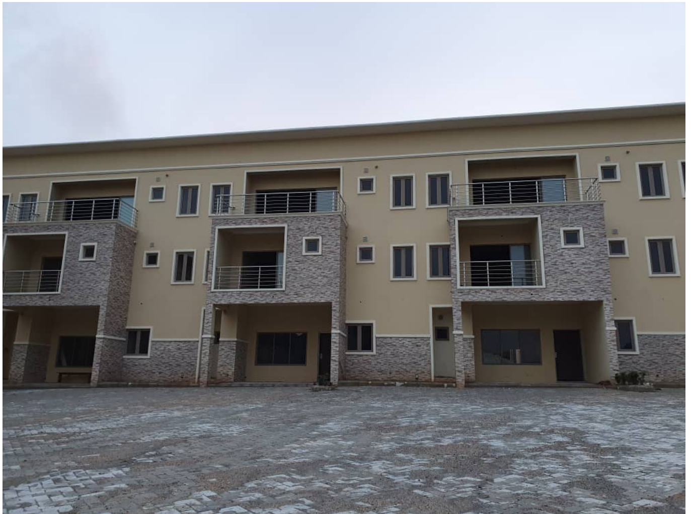
6 Unit terraces development at Katampe District Abuja
