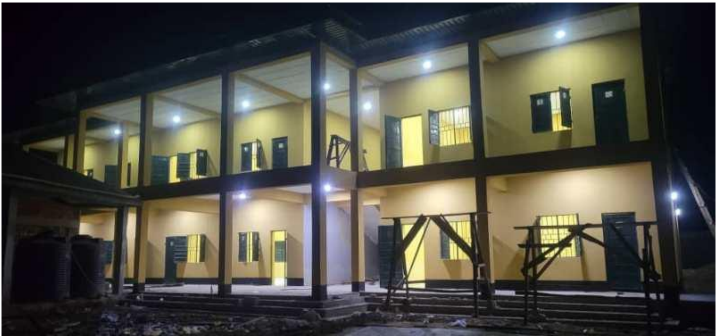
AGILE Project 2023/2023 in Zaria City: Block of 6 Classrooms
