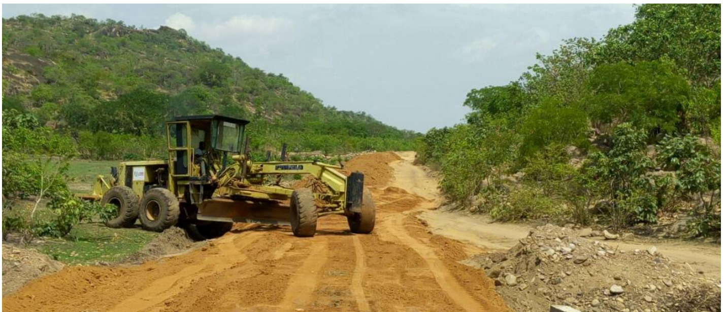
Road construction project at Kubau LGA, Kaduna State
