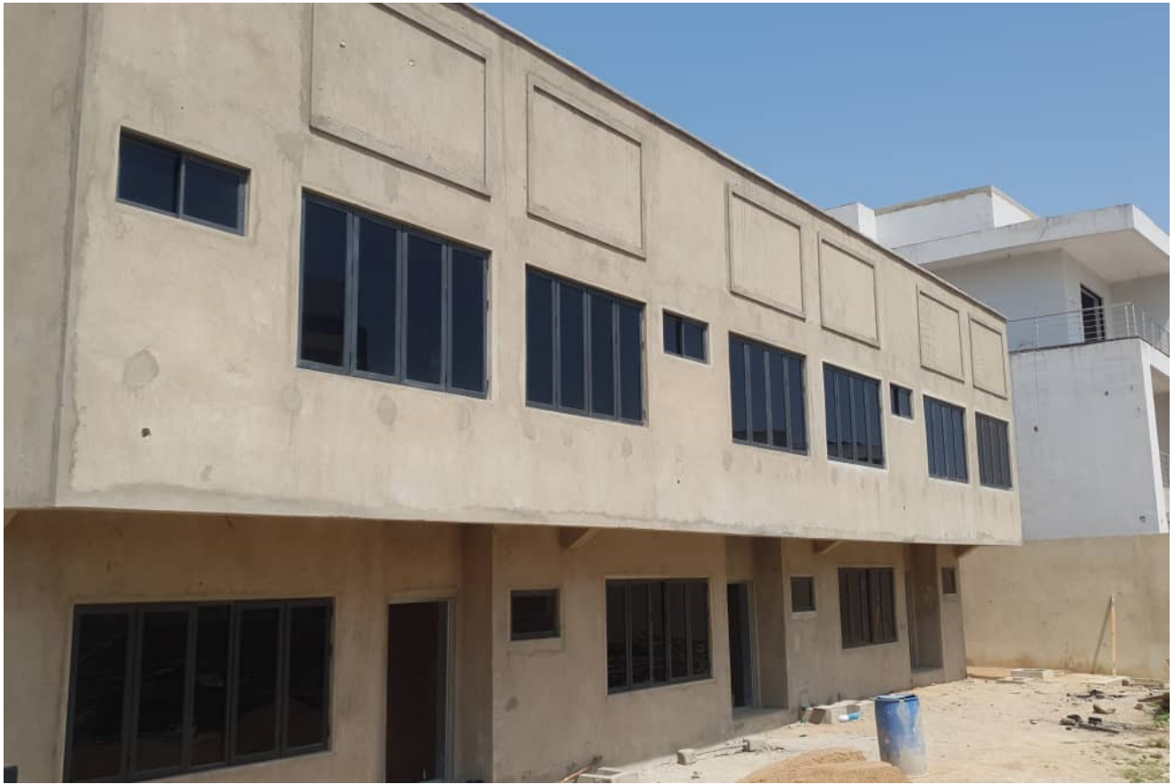
3 Terraces Residential Development at Bompai, Kano
