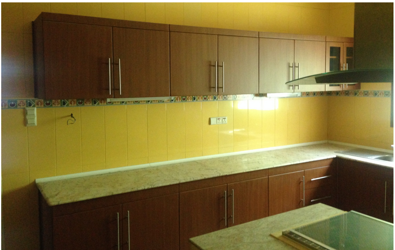
Interior Finishing & Detailing
