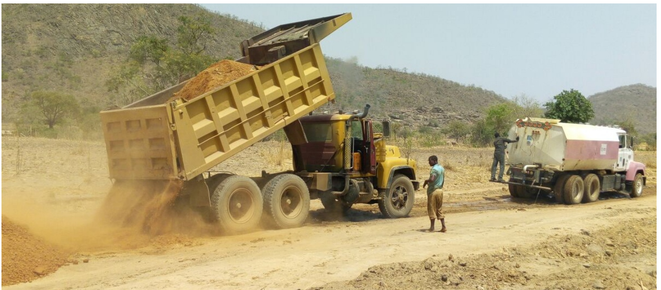
Road construction project at Kubau LGA, Kaduna State
